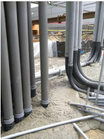
Typical flowing LCC backfill
