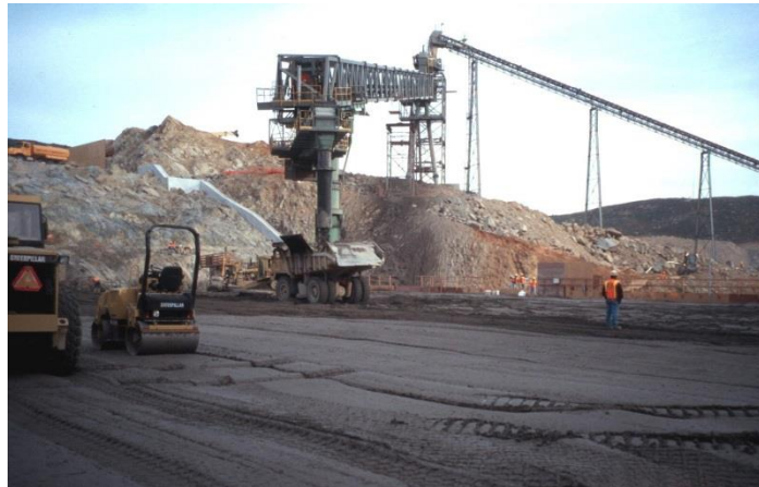
Placing RCC at Olivenhain Dam
